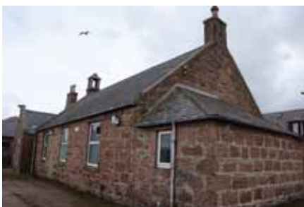
Buchanhaven School building today.
