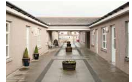
Community Service Centre - Phase 2.
